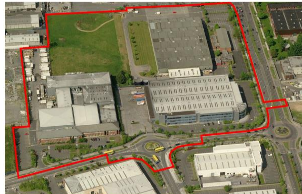
Fig. 2.2: Northward Aerial View of the overall Masterplan Site (Phase I & II) outlined in red (source: Bing Maps with Tom Phillips + Associates annotation).
