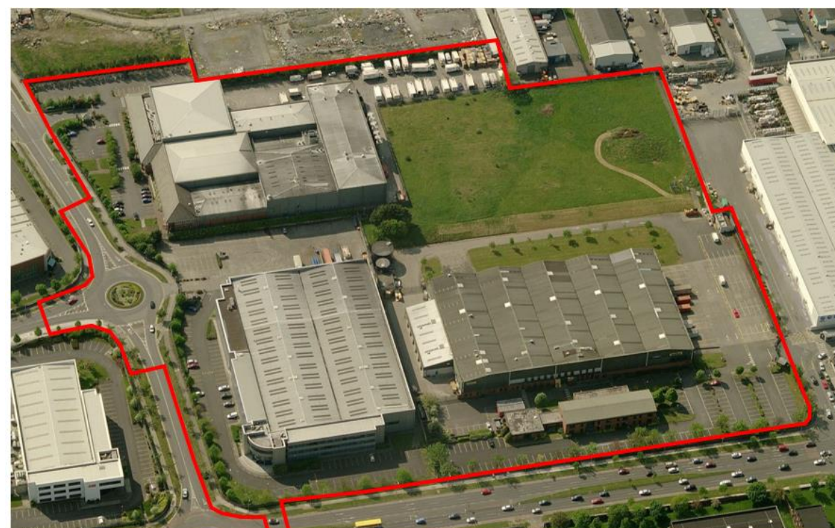
Fig. 2.3: Westward Aerial View of the overall Masterplan Site (Phase I & II) outlined in red (source: Bing Maps with Tom Phillips + Associates annotation).
